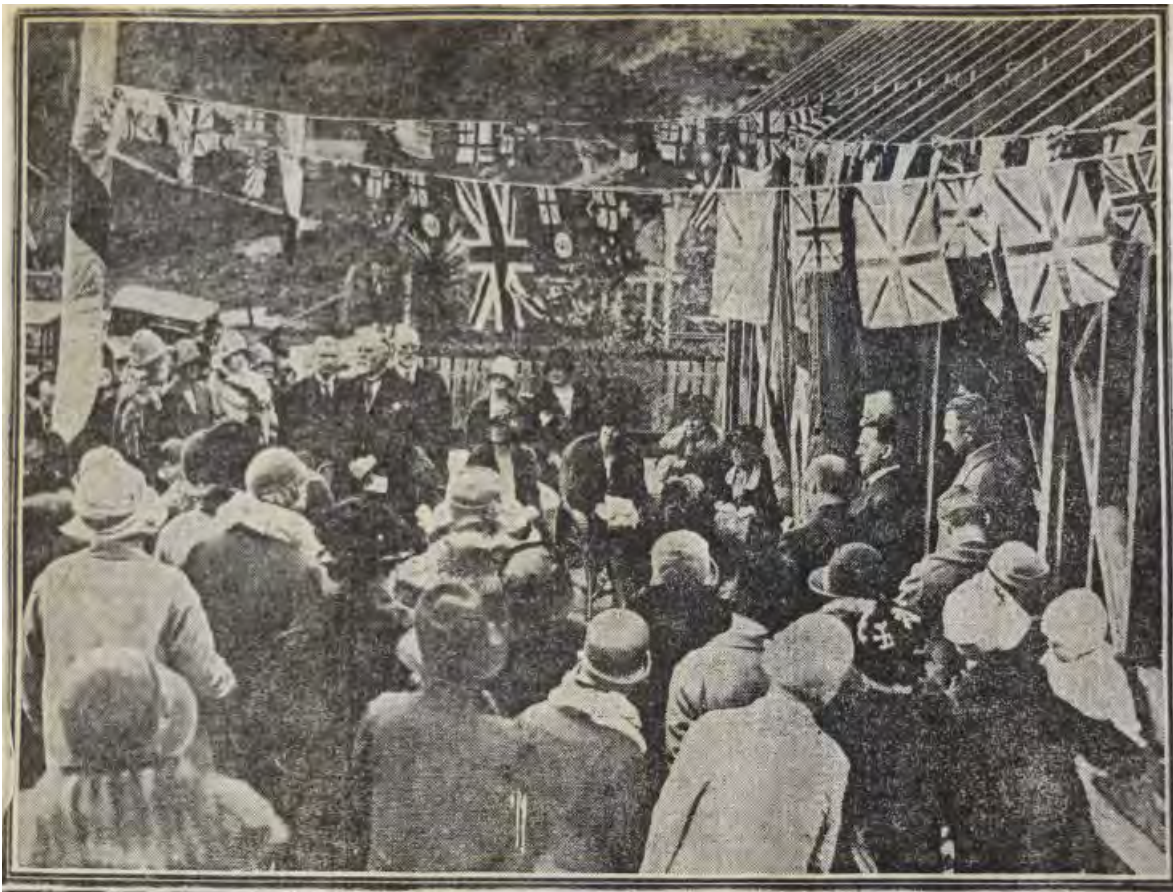
Figure 6: The laying of the foundation stone at Berhampore Kindergarten, 28 September 1928. Photographer unidentified (ATL MSY-1921)
