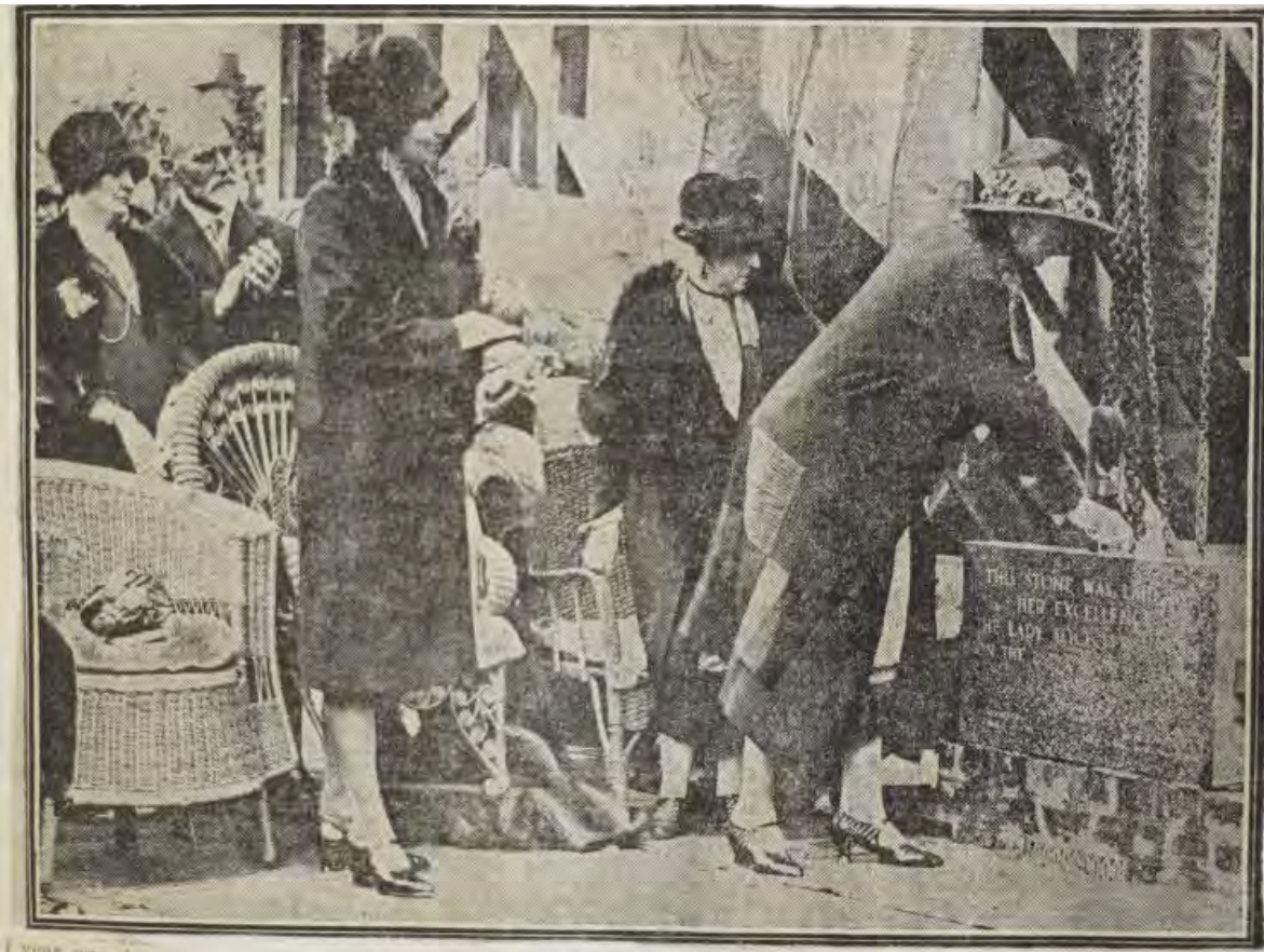
Figure 7: Lady Alice Fergusson laying the foundation stone of Berhampore Kindergarten, 28 September 1928. Photographer unidentified (ATL MSY-1921).
