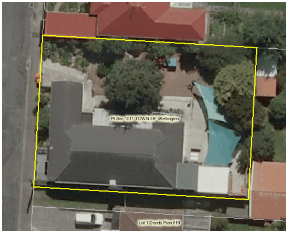
Figure 1: Aerial view of 3-5 Stanley Street, Berhampore, Wellington, showing Berhampore Kindergarten and the extent of its land parcel (Image courtesy of Wellington City Council's rates website).
