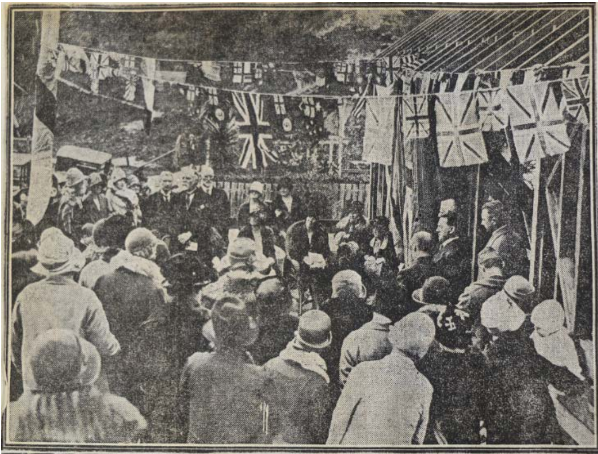
Figure 6: The laying of the foundation stone at Berhampore Kindergarten, 28 September 1928. Photographer unidentified (ATL MSY-1921)
